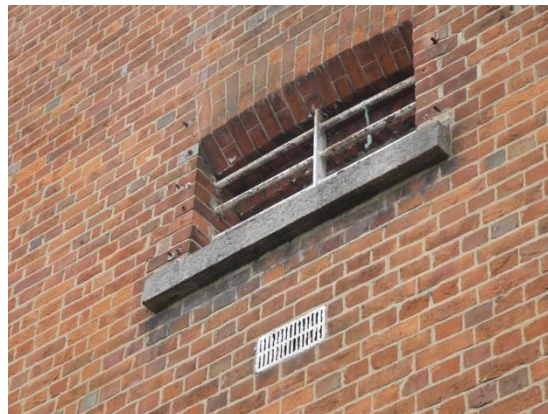
Photo 4. Example of a B wing window with mesh window grille entirely missing
