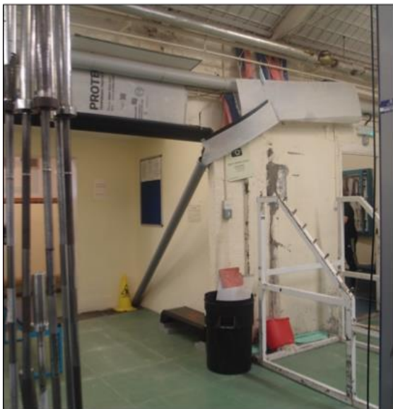
Photo 5: 2023-2024 - improvised drainage rig attempting to take leaking roof water away from the gym's operational area.
