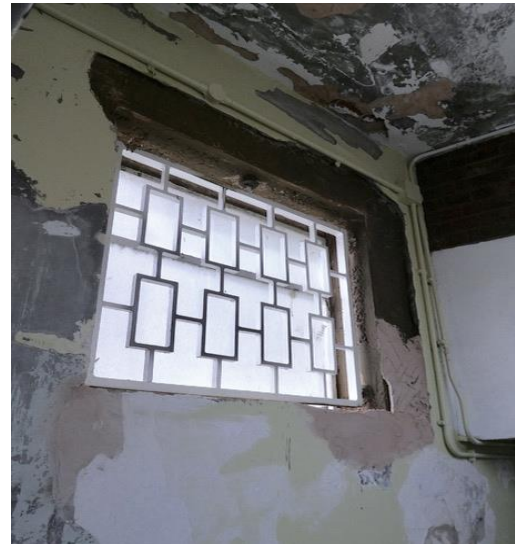
Photo 10: Effects of water ingress A wing corridor – repair started but then stalled
