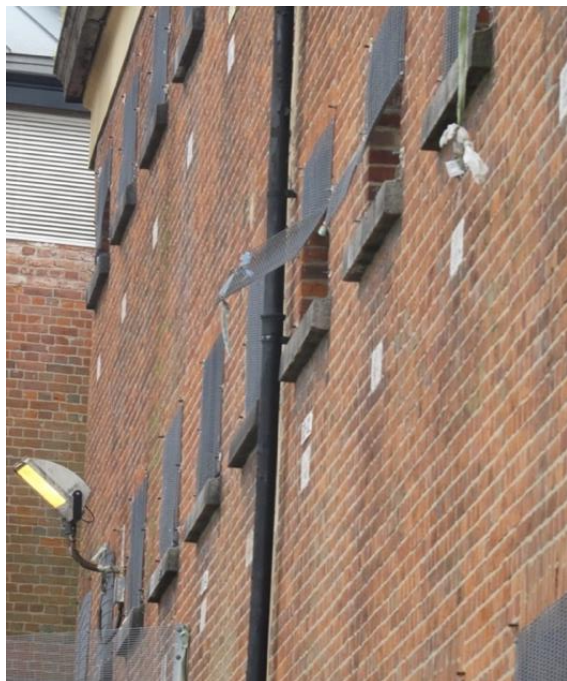
Photo 3. B wing mesh window grilles bent outward by prisoners creating potential access for drones
