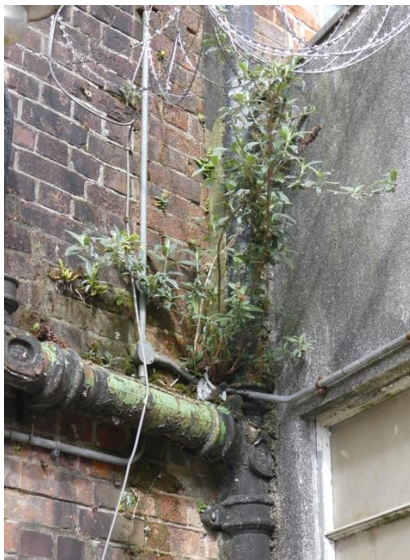
Photo 9: Vegetation growing on A wing wall junction as a result of leaking roof gutter lacking end-stop above
