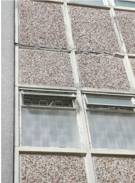
Photo 11. Deteriorating concrete framing of the education and reception block
