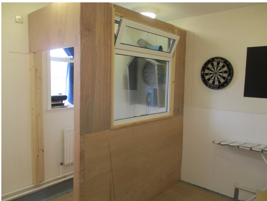
Phone booth under construction
