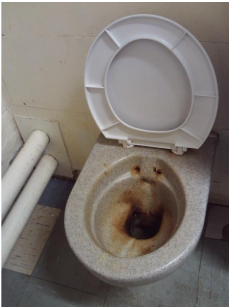
C wing cell toilet
