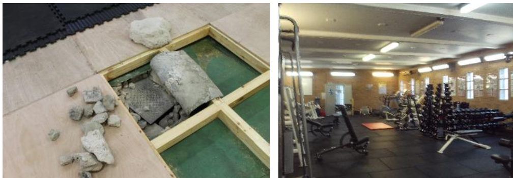
Damaged gym floor before refurbishment (left) and gym after refurbishment
