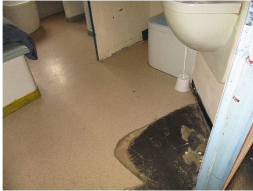
Damaged cell flooring (left) and leaking toilet
