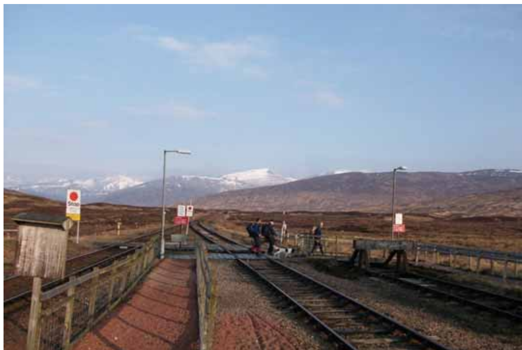
A private footpath crosses the West Highland line at the user-worked level crossing (UWC) at Corroun station on Rannoch Moor.
