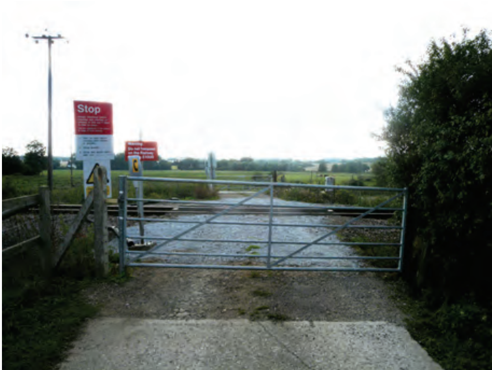
Sewage Works Lane level crossing, a user-worked, private level crossing near Sudbury, Suffolk. Credit: Rail Accident Investigation Branch
