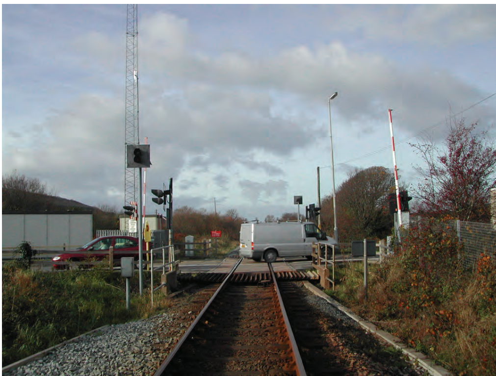
Llanbadarn automatic half-barrier level crossing (locally monitored), near Aberystwyth, seen from the train driver's perspective. Credit: Rail Accident Investigation Branch.
