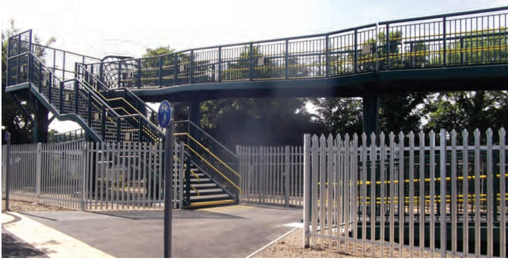
Footbridge at Fishbourne, East Sussex, built to provide a step-free replacement for the public footpath user-worked level crossing. The local authority and Network Rail are co-operating to seek permanent closure of the level crossing. Credit: Network Rail.
